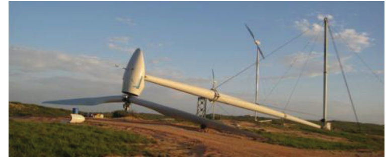
Figure 33: Wind turbines at Coral Bay are able to be tilted down during cyclones.
