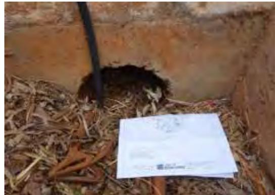
**Photo 10 Blocked culvert**
