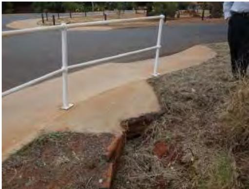
**Photo 9 Blocked Culvert**
