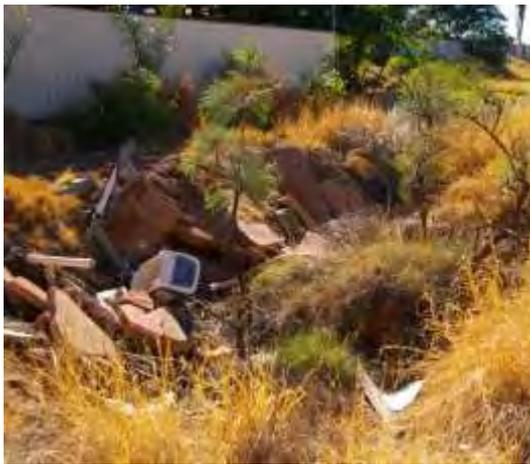
**Photo 3 Uncontrolled infill of drainage reserve**
